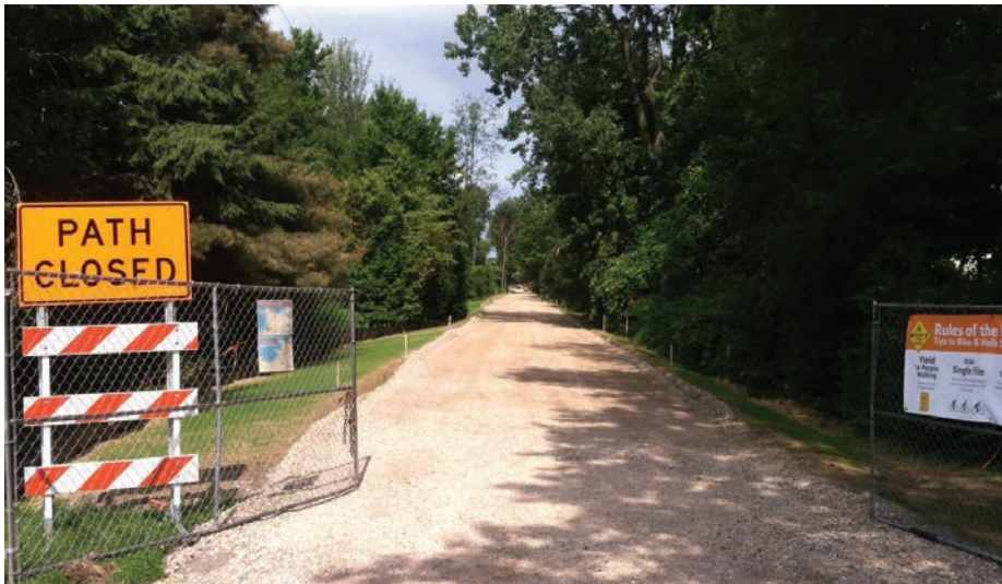
New sub-base almost ready for new pavement.
