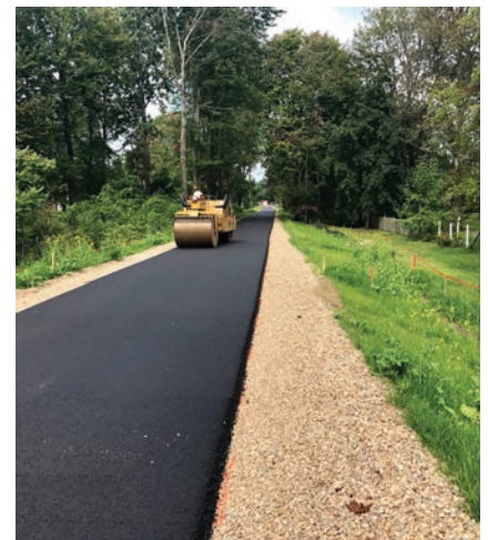
Paving the new 11" wide path.
