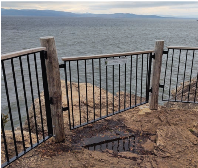
The view from Rock Point is improved with new safety fencing.
