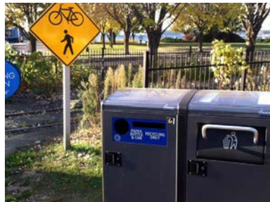
Summer '14 Big Belly trash compactor installation at Waterfront Park.
