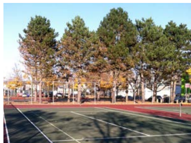
Tennis court renovations at Roosevelt Park, summer '14.
