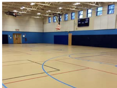
Renovation of the gymnasium floor at the Miller Community Center.
