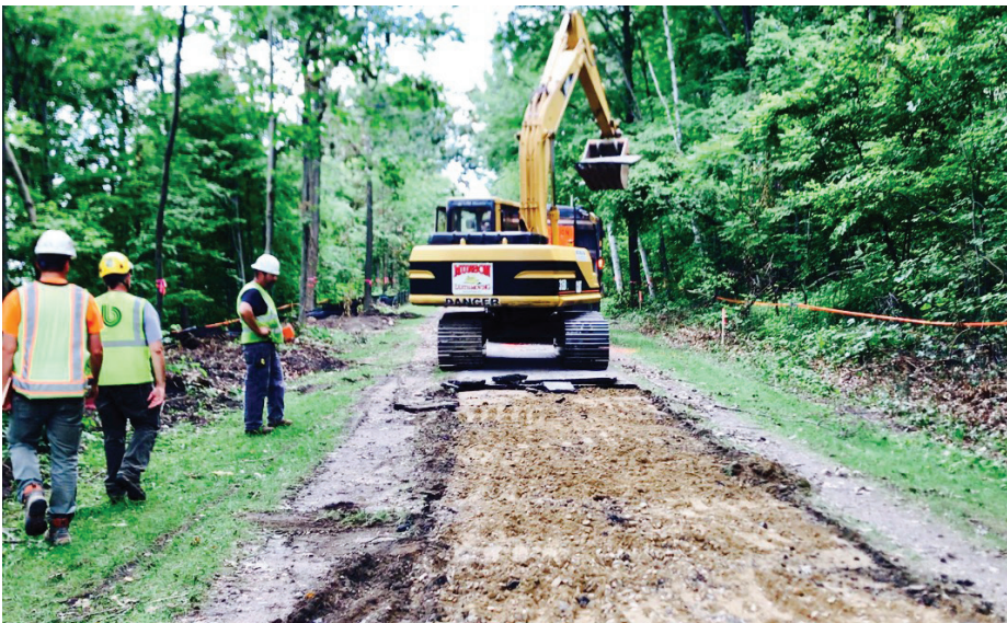
Construction crews remove the old path.
