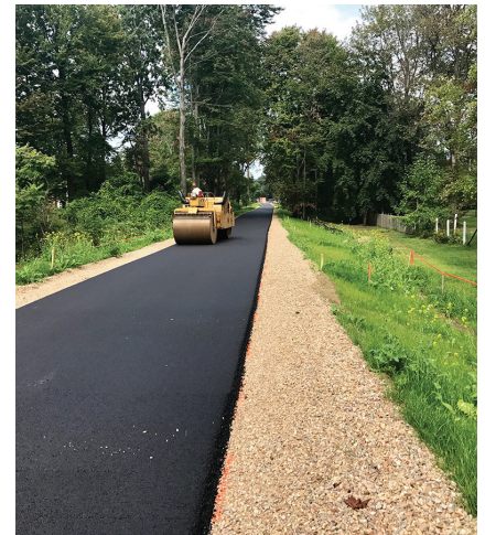
Paving the new 11" wide path.
