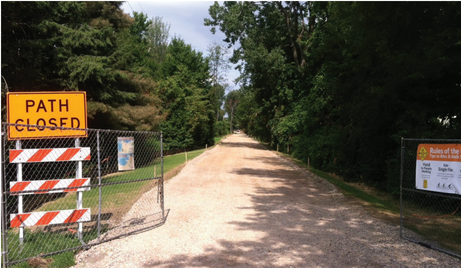
New sub-base almost ready for new pavement.
