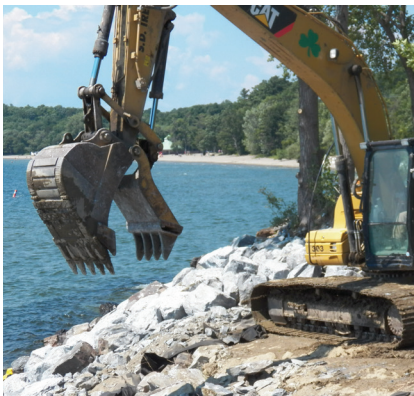
Shoreline stabilization near new Bike Path route.
