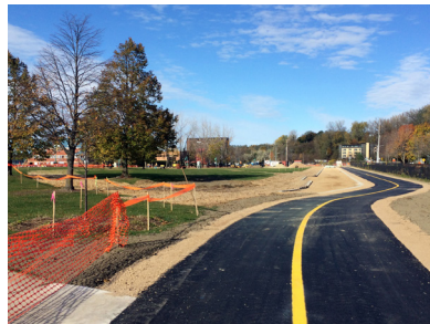
November '14 reconstruction of the Bike Path through Waterfront Park.
